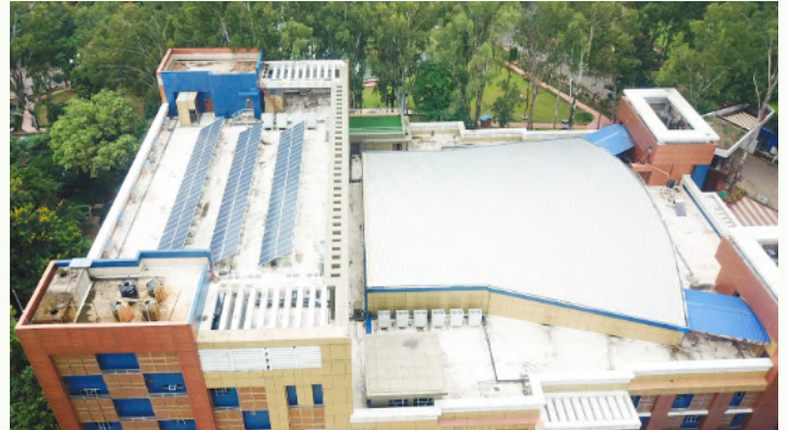
View of rooftop Solar Panels at Darbhanga House CCL HQ
