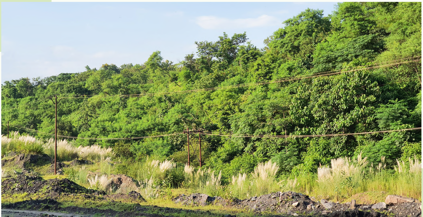
View of Plantation over embankment at Rohini OCP
