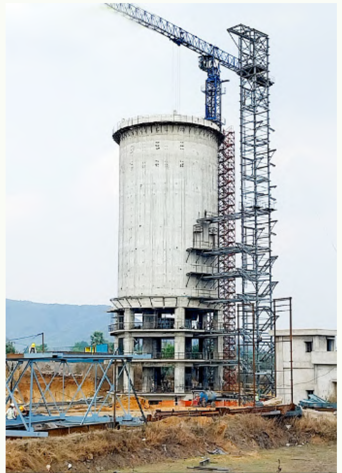
Under-construction CHP-Silo at North Urimari OCP
