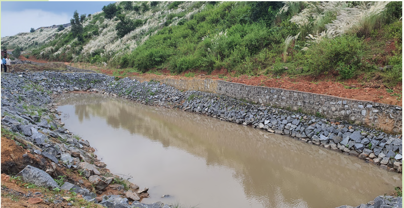
View of Settling Pond near toe of OB Dump at Amrapali OCP
