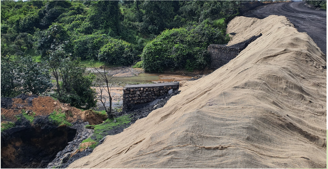
Jute Netting near streams at Amrapali OCP
